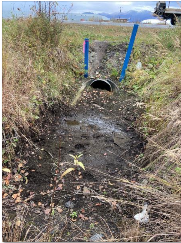
SW6. East view of culvert through Minnesota Drive
