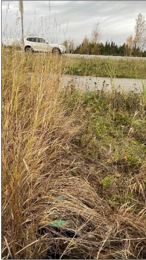
SW2. South End of Culvert under Raspberry Road
