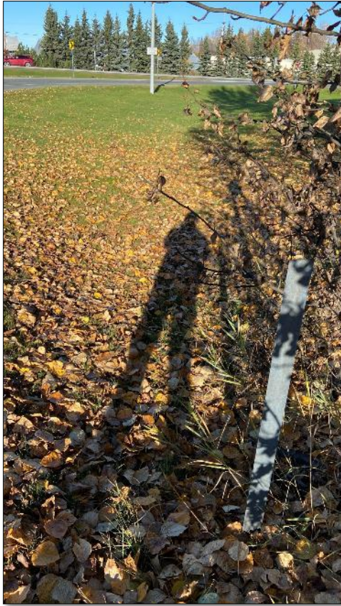
SW13. Looking north at culvert under bike path along International Airport Road onramp
