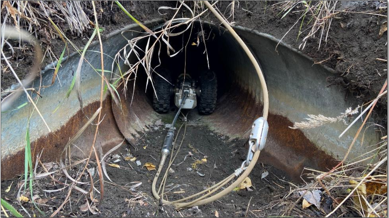
SW1. South end of culvert under Raspberry Road
