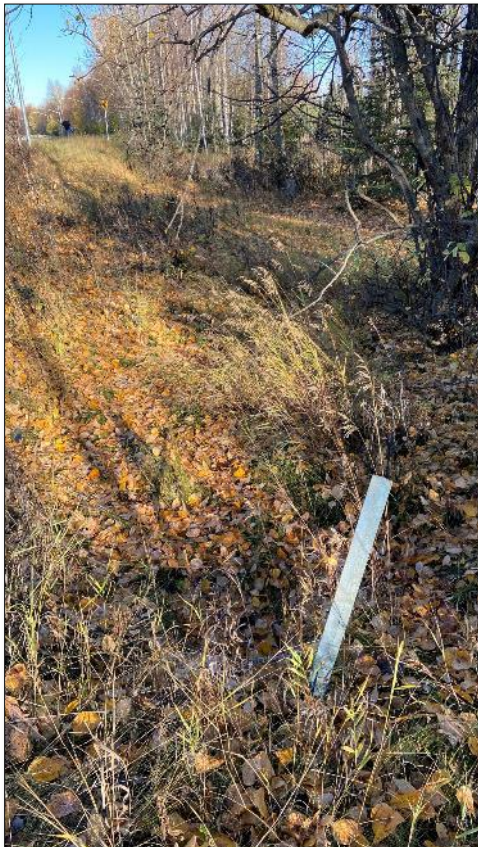
SW14. Looking northeast at culvert under Collins Way
