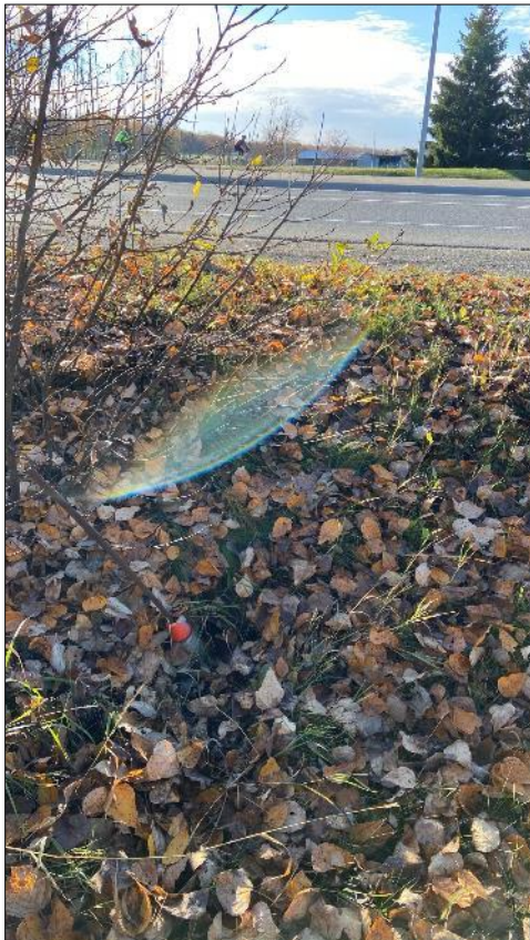
SW12. Looking southwest at small culvert under Jewel Lake Road
