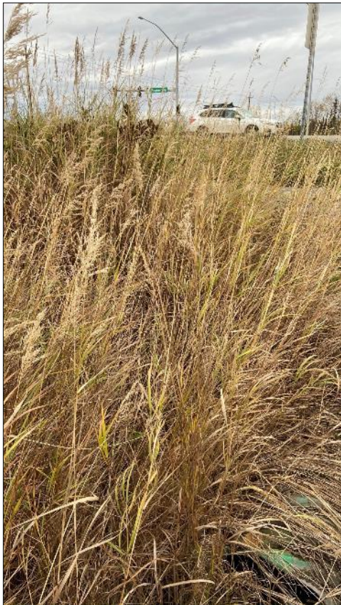
SW3. South End of Culvert under Raspberry Road
