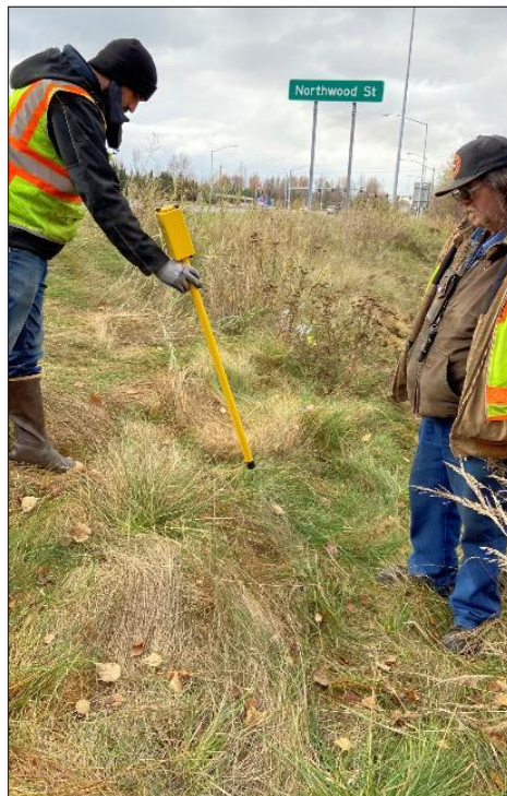
Inset 3. MOA staff detecting the north end of the culvert under Raspberry Road
