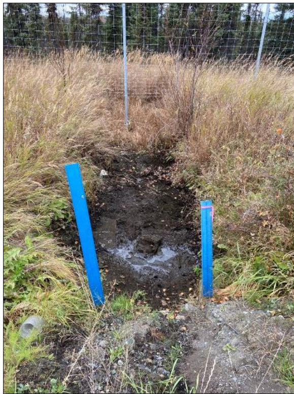
SW6. West view on top of culvert through Minnesota Drive
